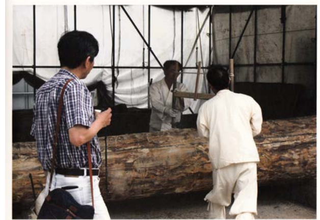
Figure 7. Carpenters in Korean dress using traditional tools to prepare domestic pine trees (Source: CHA 2011).
